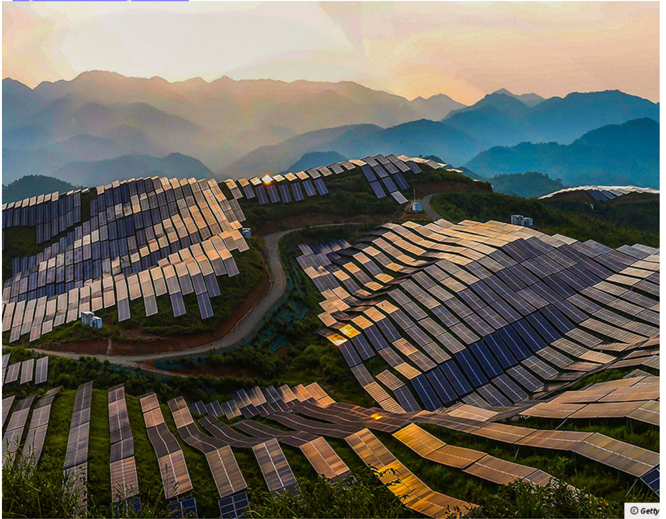
Renewables: Around the world, solar panels, such as these at the Xinyi power station in Songxi, China, produce huge volumes of clean, free electricity.
